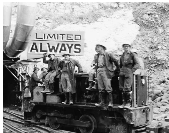
Workers pose before going on shift in the Tooma-Tumut tunnel – National Archives of Australia
