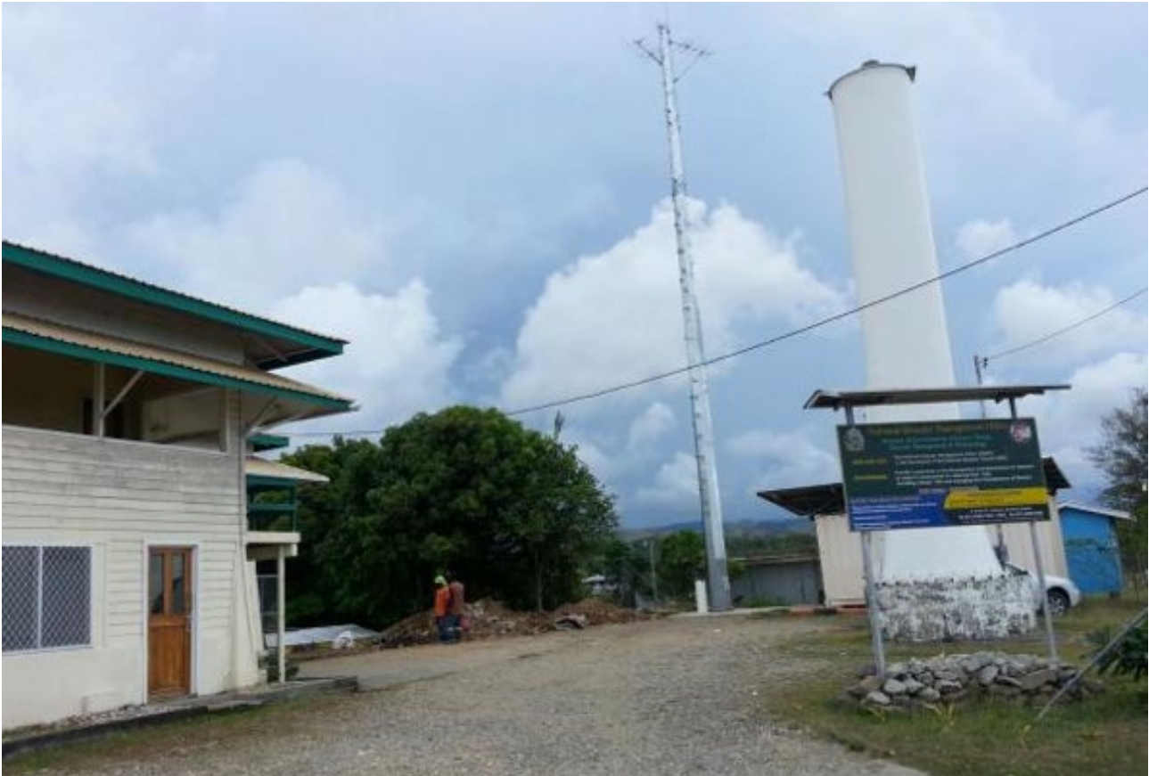
Figure 1: The backup receiver tower at the National Disaster Management Authority office. Photo by Joys Eggins, October 2012
