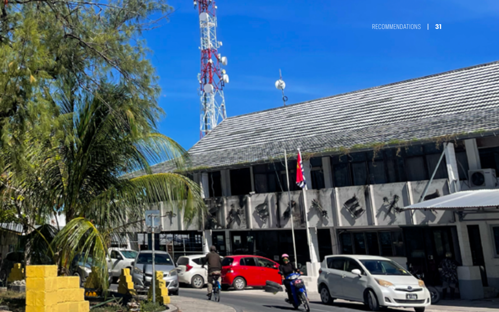
Telecommunications infrastructure, Bairiki, Tarawa. (Vicki Kerrigan)
