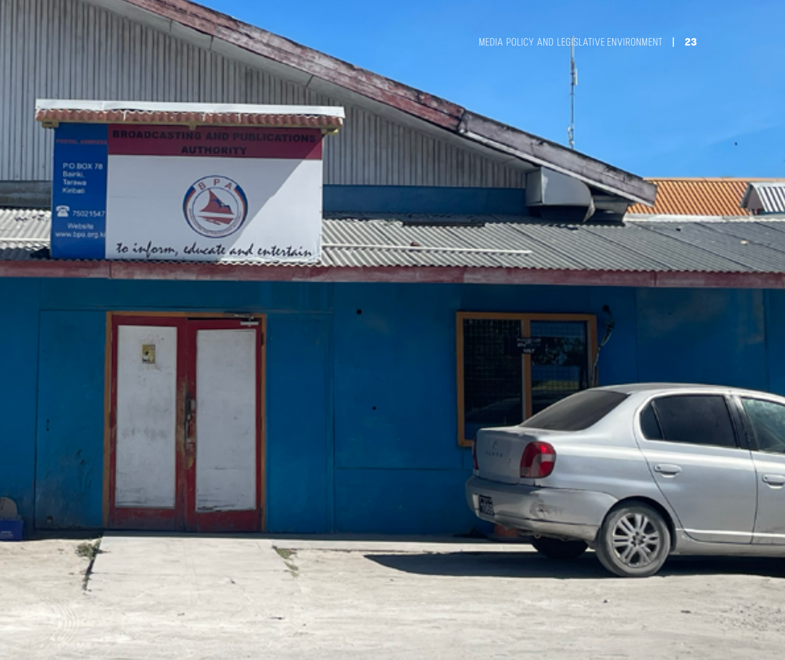
Broadcasting and Publications Authority (BPA) building, Bairiki, Tarawa. (Vicky Kerrigan).
