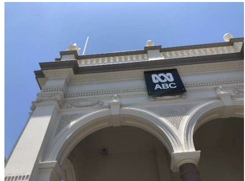
Figure 41: The upper portion of the front façade, including the entablature and cornice.
