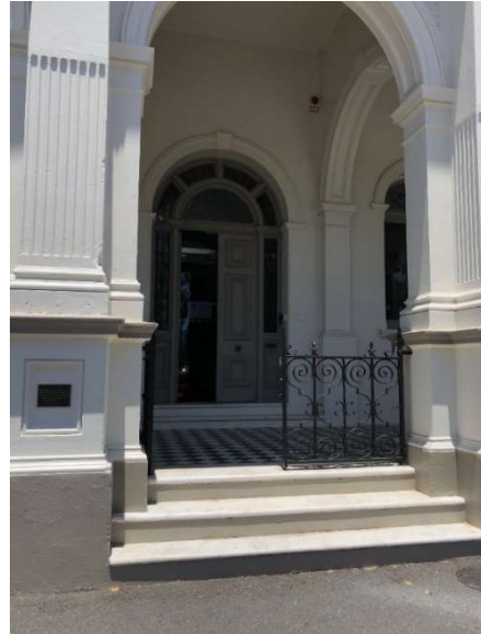
Figure 35: Front steps and wrought iron gated entry along the front façade.
