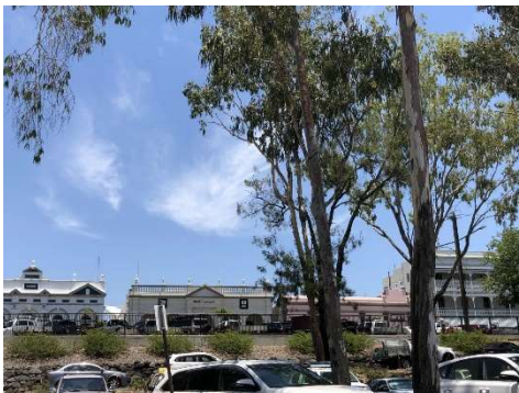
Figure 29: View of the ABC Radio Studios building looking southwest from the riverside parkland adjoining the Fitzroy River.
