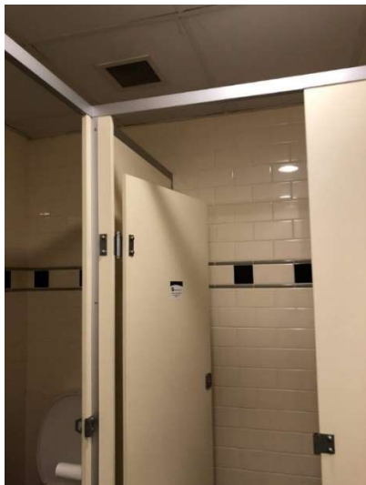
Figure 97: Bathroom, noting later fitout and later ceiling.
