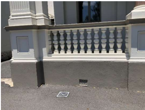
Figure 40: The front façade plinth.
