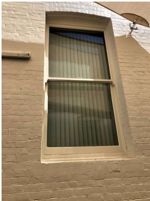
Figure 46: Detail of original side elevation window.
