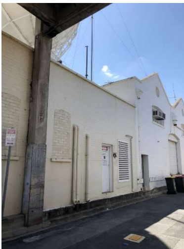
Figure 50: View of the rear elevation showing brick infilled window opening to the eastern side of the elevated substation.
