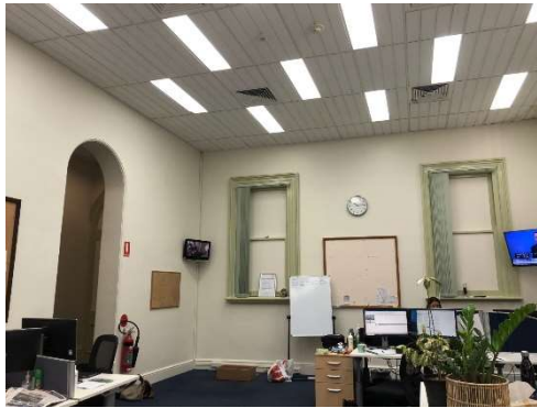
Figure 77: Broadcasters room, noting arched opening to the left and infilled window frames.
