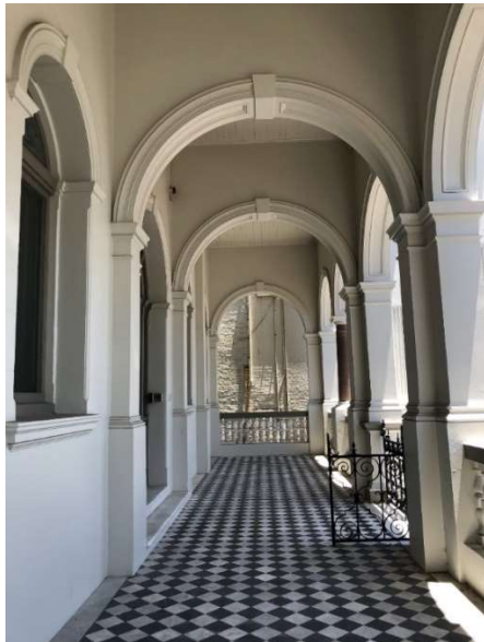
Figure 36: View along the front verandah, looking northwest.
