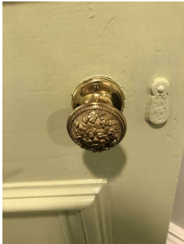
Figure 71: Early door hardware.
