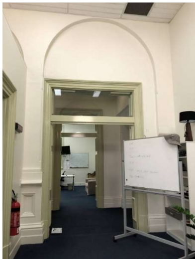
Figure 73: View back towards the hallway from the journalists room, noting door opening and associated joinery.
