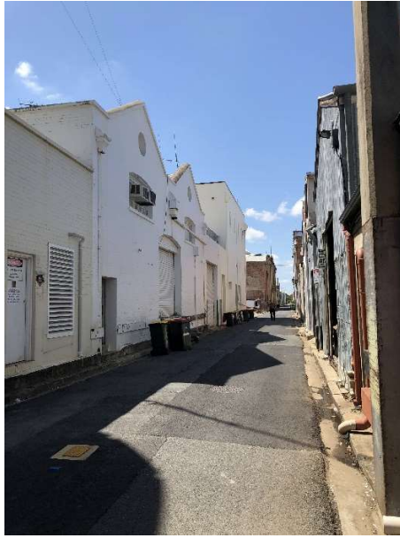
Figure 31: View along Quay Lane at the rear of the building looking southeast.
