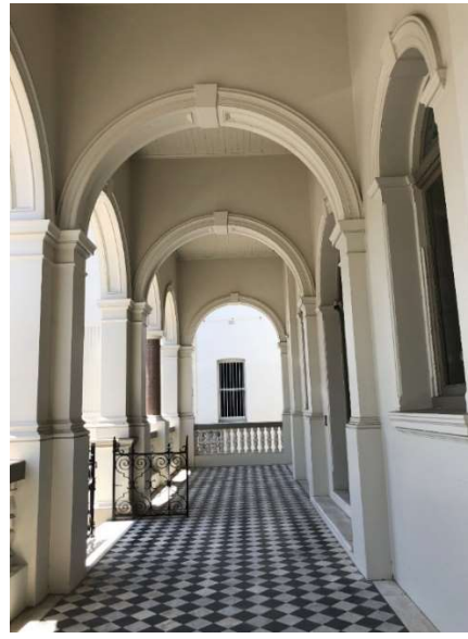
Figure 37: View along the front verandah, looking southeast.
