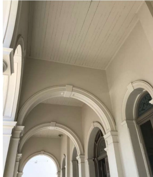
Figure 39: Front verandah soffit.
