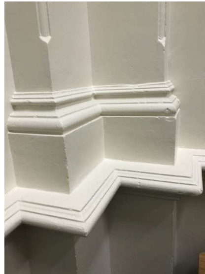
Figure 84: Wall and dado detailing to the TV editing room.
