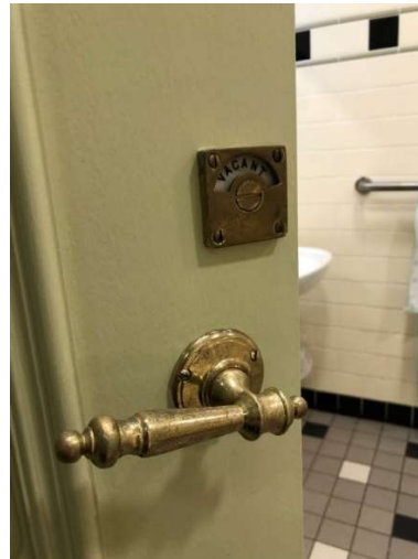
Figure 96: Bathroom door, noting joinery.
