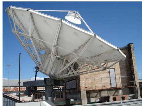
Figure 53: Satellite dish on the roof of the rear addition. (NBRS + Partners, June 2011)
