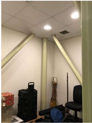
Figure 95: Rear storeroom, noting cross bracing along the walls.
