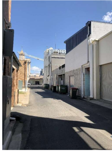
Figure 32: View along Quay Lane at the rear of the building looking north-west.
