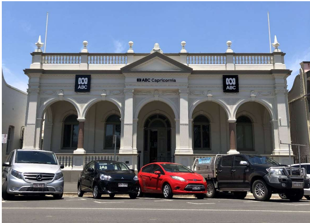
Figure 33: View of the front façade of the ABC Radio Studios building from Quay Street.
