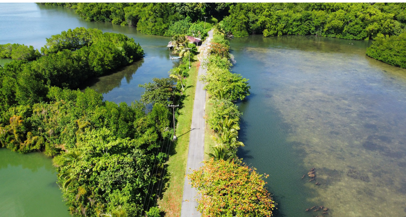
The Temwen Access Road in Nihkawad, Pohnpei. (Hamish Wyatt/World Bank)
