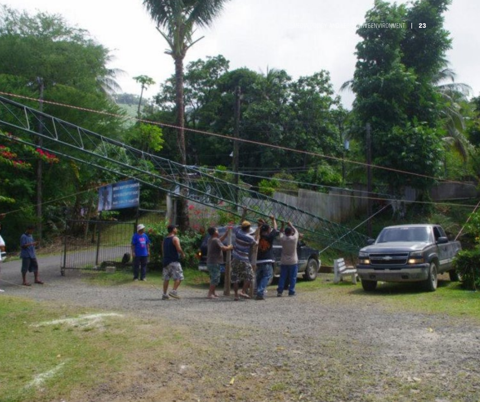
Erecting Bible Baptist Radio's new tower in 2013. (Facebook: Bible Baptist Radio Station 88.5FM)
