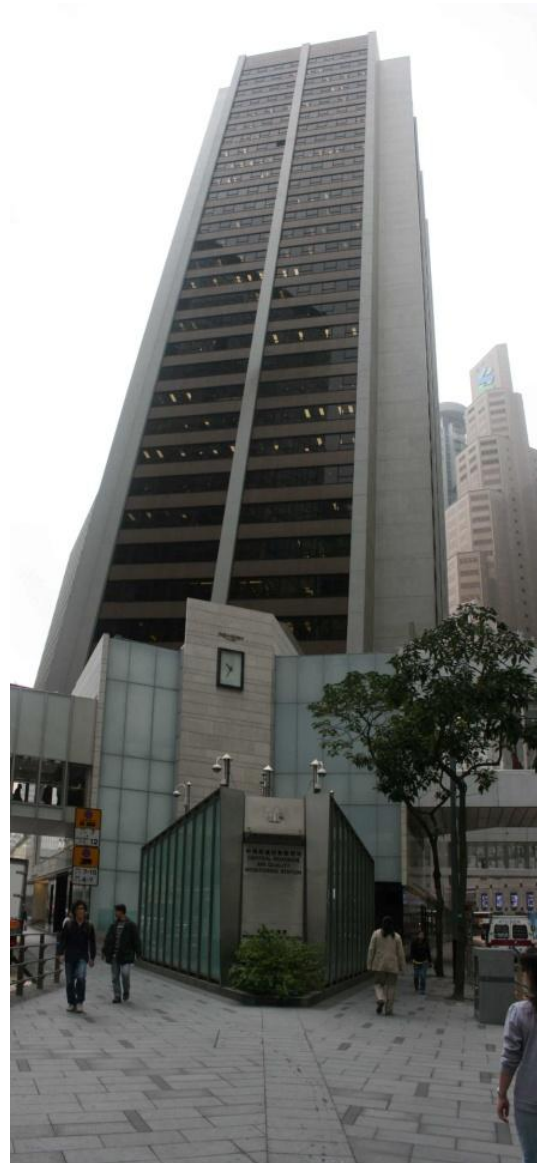
Figure 08: Alexandra House , photo by author
