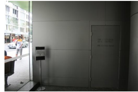
Figure 53: Fire control room, photo by author
