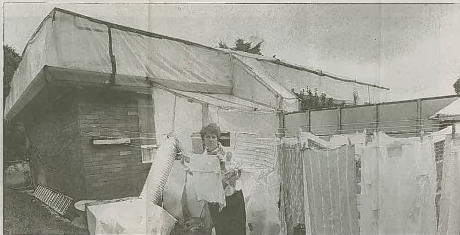
THE CANBERRA PROGRAM: Mrs Frances Christie hangs out the washing in her back yard in Pearce in 1989, practically surrounded by asbestos-removal equipment. The roof is shrouded in plastic and in the foreground is a dust-extracting machine.
