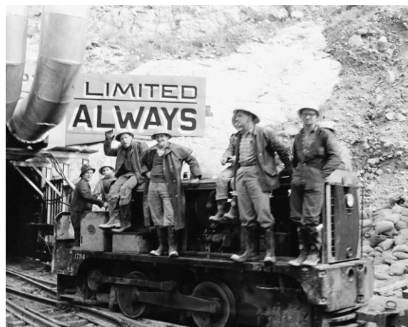
Workers pose before going on shift in the Tooma-Tumut tunnel – National Archives of Australia
